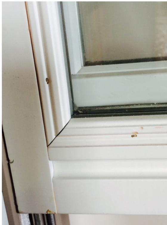
9) **Figure 9** – In order to determine the size of your window, you can do the following: 1) look for the head label on your window(s) (see Figure 3) containing a “Size” number (Not every window will have a head label.); or 2.) measure the “daylight opening” of one of the sashes (the length and width of the glass in inches) as indicated below.
