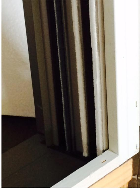
**Figure 6b** – Example of Lower Frame (sash closed) and Sill from Exterior; Note – Sash may be open or closed:
